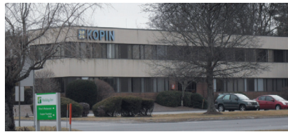
For Lease, ext. 323 Myles Standish Park, Taunton, MA 25,000 Industrial Building Clean Rooms
